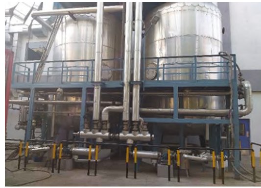
Blenders for the production of specialty oils at our Taloja Plant
