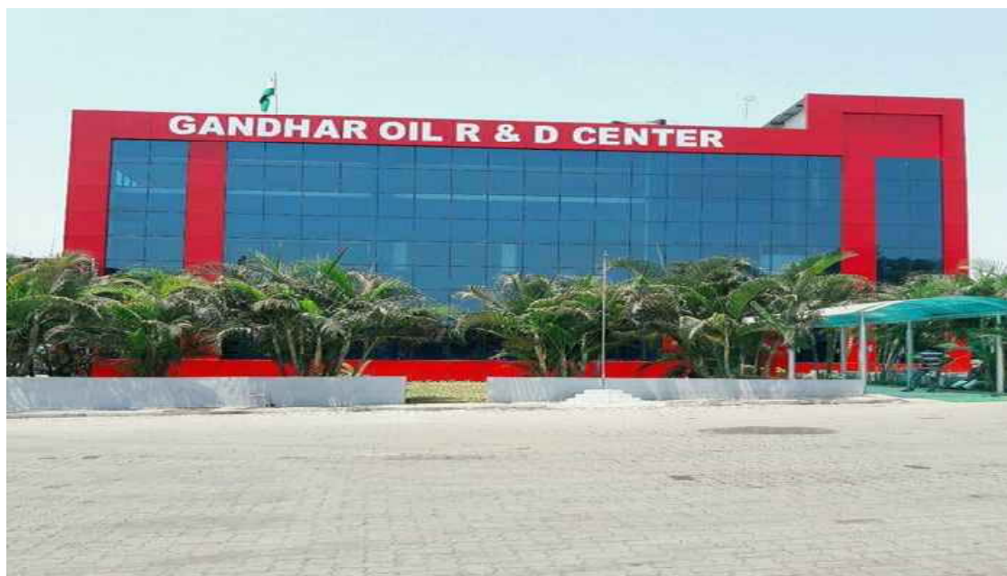
R&D center at our Silvassa Plant
